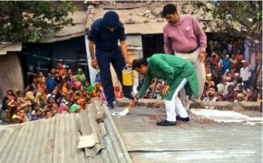
Figure 1: Slums being painted with solar reflective paint by Ahmedabad Municipal Corporation (AMC) in 2020 (top). Former Ahmedabad Mayor Gautam Shah painting a cool roof with white paint in Ahmedabad, India, in 2017 (bottom).
